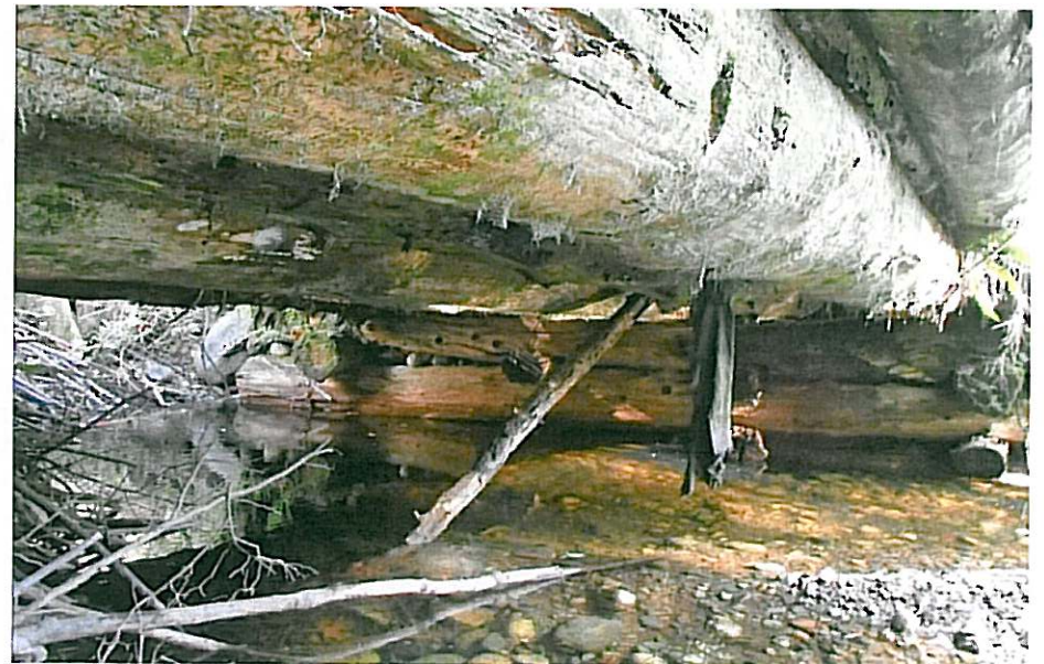
CK-2263 Left Abutment
