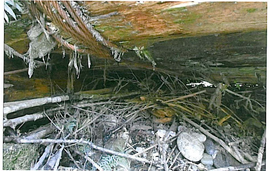
CK-2263 Right Abutment
